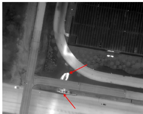
Figure 19. Leakage in an aerial thermal image
