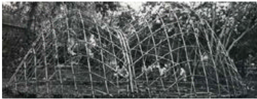
Finished grid shell
