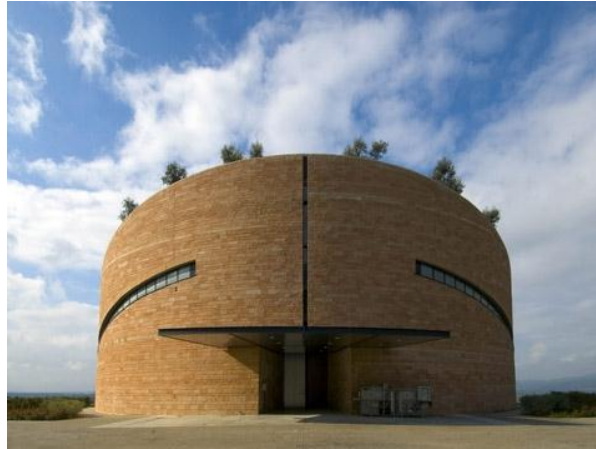
Cylinders in architecture (creating nodal points): Petra Winery in Suvereto , Italy by Mario Botta
