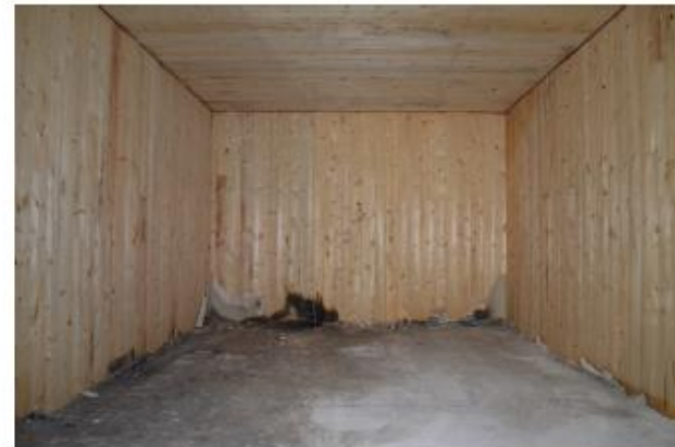
Room after drywall removed following the three-hour test
