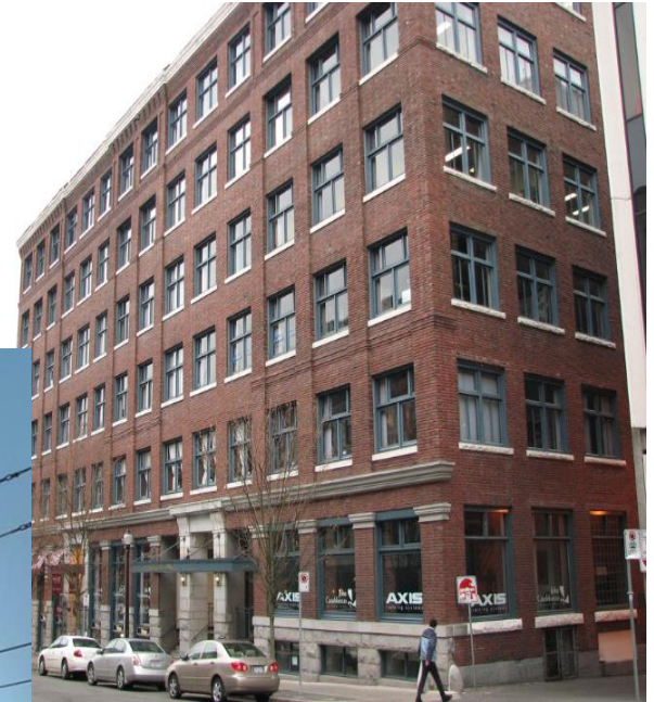
Leckie Building, Vancouver, BC (c. 1908)
