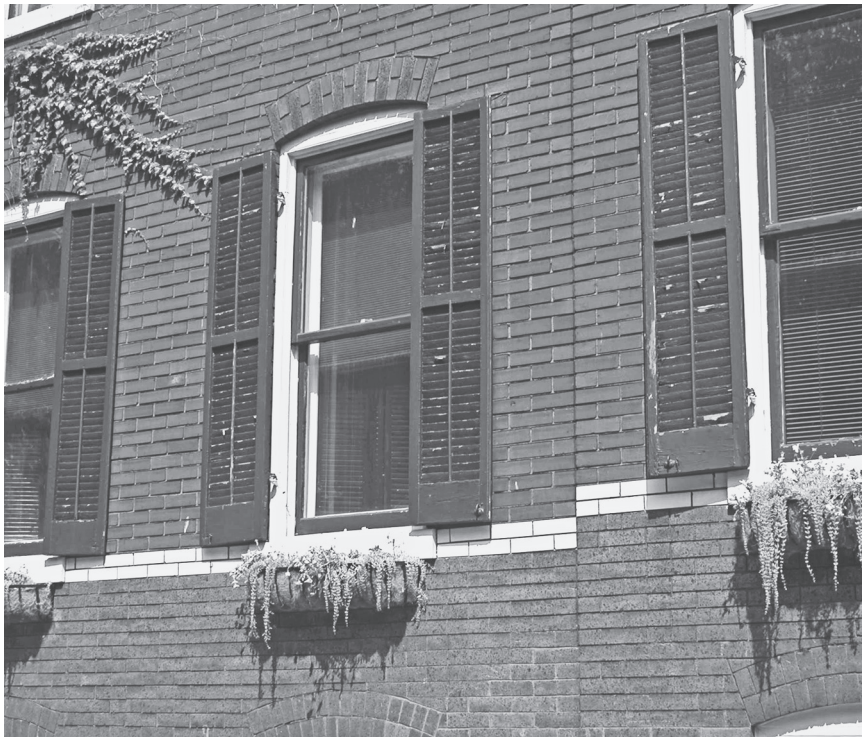
FIGURE 1.2. Prior to air-conditioning, buildings were equipped with features to take advantage of natural ventilation, such as operable sash, louvered shutters (a), and transom lights (b).
