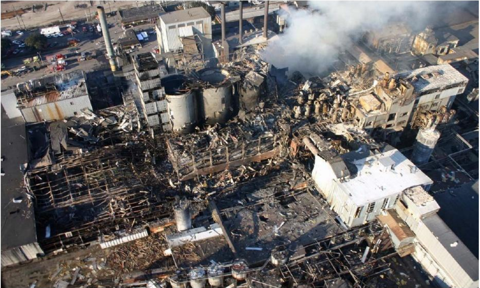
Figure 1. Aerial photograph of Imperial Sugar Port Wentworth facility after explosion.
