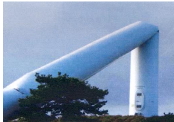
Global buckling of a wind turbine tower
