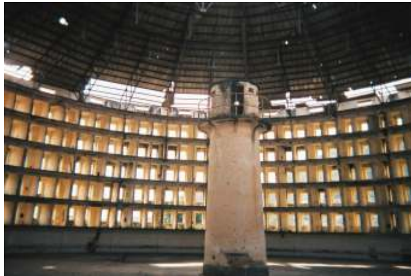
Figure 7.6. The Presidio Modelo Prison, Cuba, built between 1926 and 1928 was based on Bentham's panopticon design. (Photo courtesy of Friman/Wikimedia Commons)
