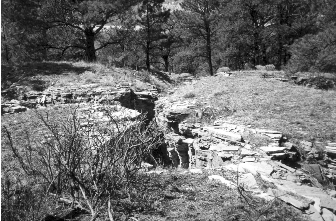
Figure 16. Fractures in Minnekahta Limestone, apparently extending down through the entire thickness of the formation, locality B, Cascade Springs, Stop 4.
