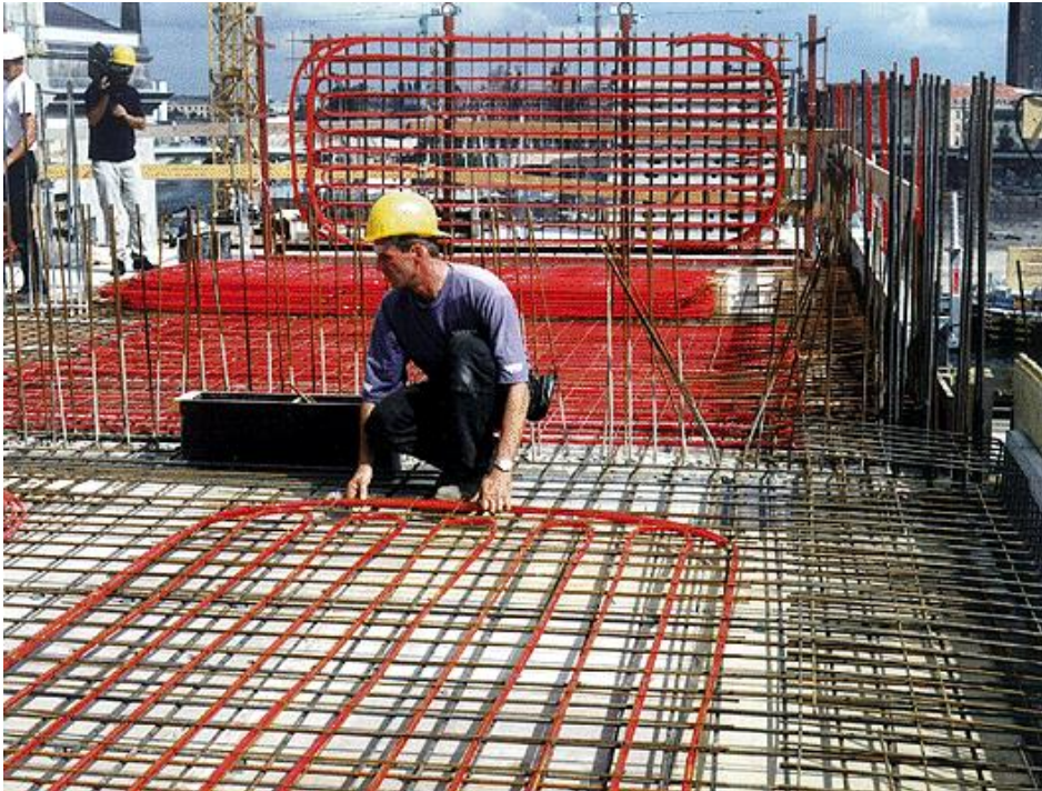
Horizontal loop systems within/beneath slabs
