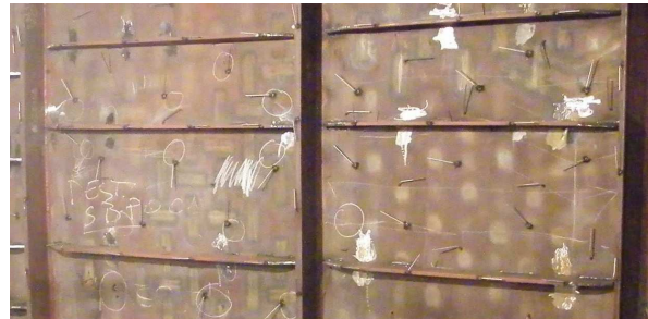
Fig. 1. Two wall segments with studs welded in place and bend.
