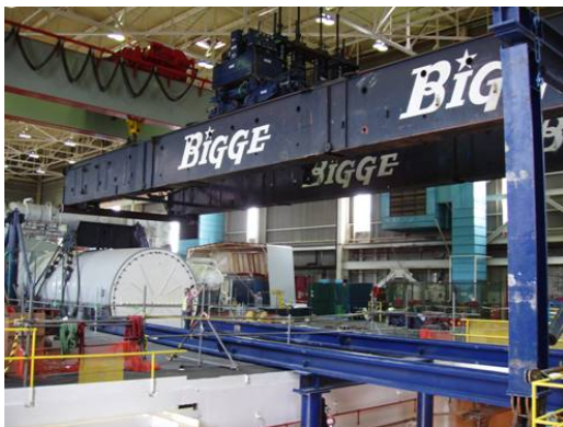
Figure 2 - Runway girders being erected
