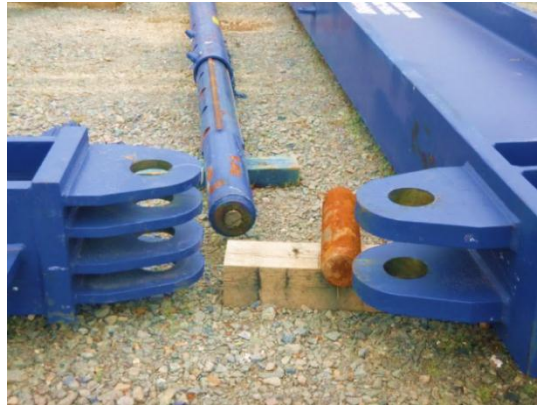
Figure 32 – Lower connection of the upper NE column.
