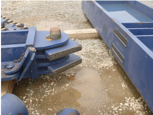
Figure 28 – Lower connection of the NW column.
