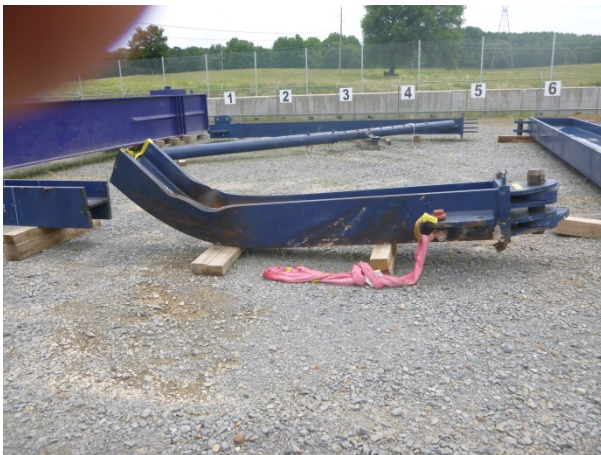
Figure 24 – Lower NW column
