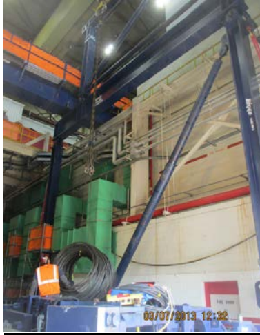
Figure 7 – North frame being erected
