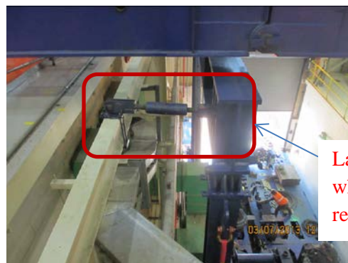
Figure 5 - Lateral brace installed
