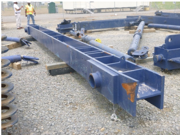
Figure 36 – East end of the top header beam
