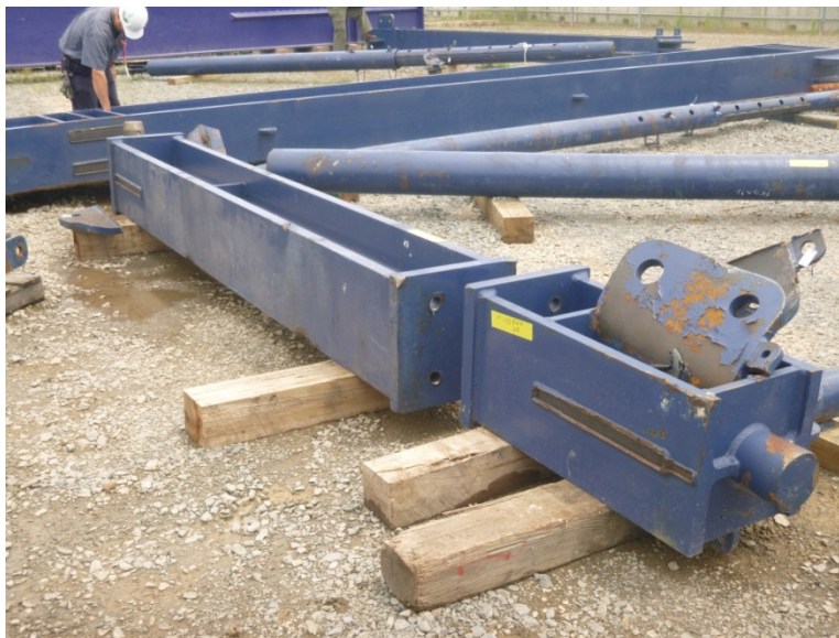
Figure 30 – Top pin connection of the upper NW column
