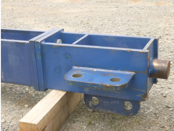
Figure 22 – Bottom pin of lower NW column
