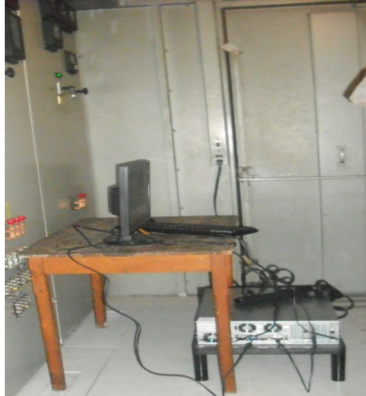
Figure 7-18 Wireless IED installed close to relay panel in 27.6 kV substation
