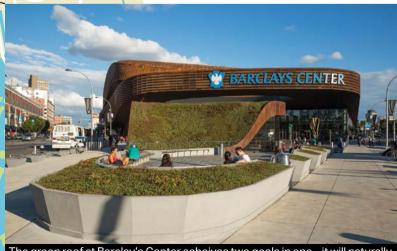
The green roof at Barclay's Center acheives two goals in one – it will naturally treat rainwater, relieving pressure on New York's sewage system, and it muffles sound enhancing the acoustics of America's boldest new arena.
