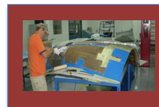
Structural Component Repair
