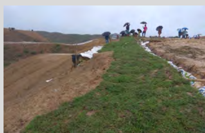
Planting grass on slopes to avoid water infiltration.
