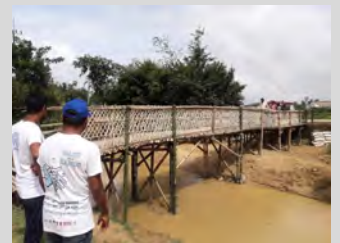
Completed 24-meter bridge in Camp 9.
