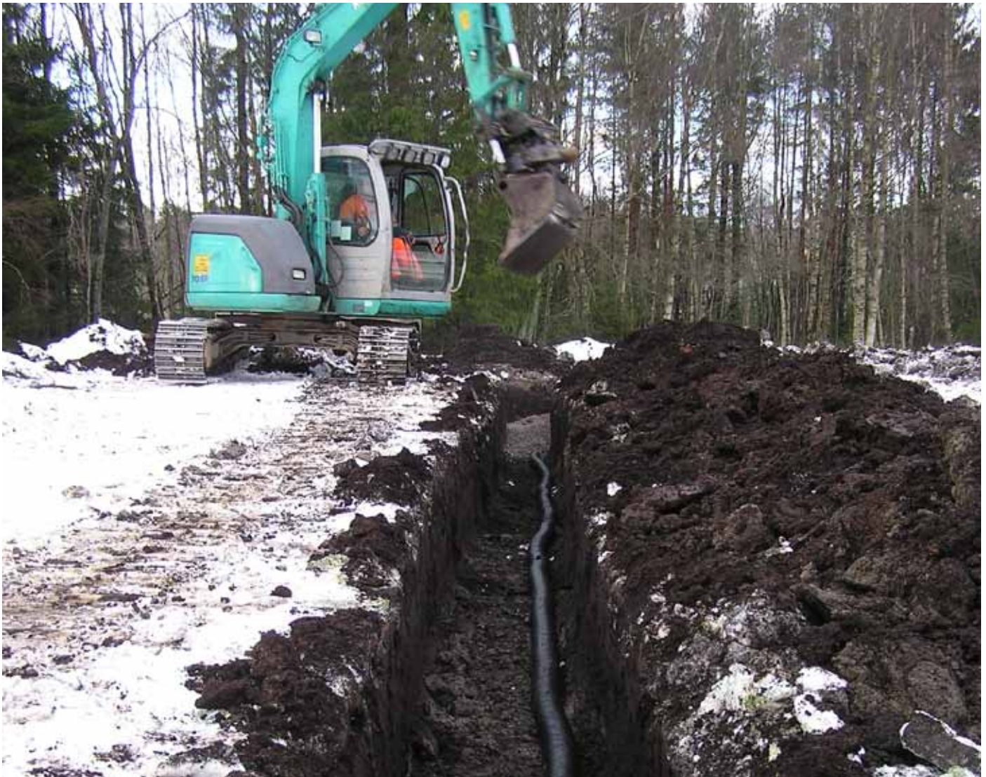
Photo 1. Drain pipes lower the soil water table. Photo: Agnar Kvalbein.
