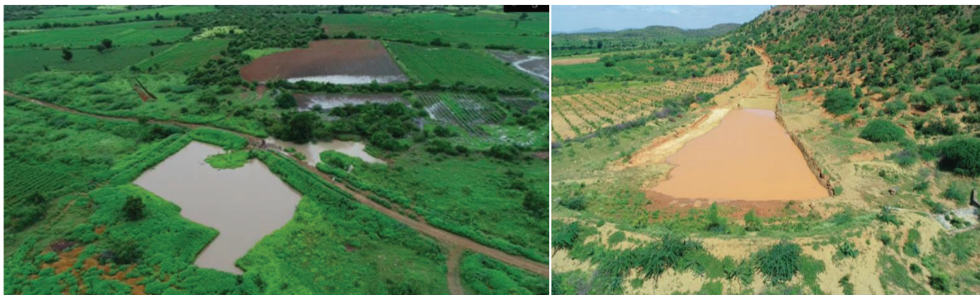
Percolation tank and sunken pits built on a stream in Patnikota village of Kurnool district. (R) Desilted percolation tank in the downstream village of Ayyavaripalli in Anantapur district, Andhra Pradesh state, India.
