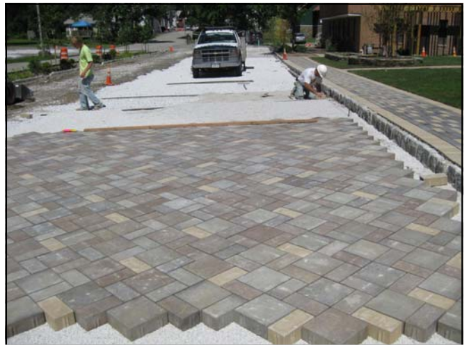
At work on installing the pervious pavers.
