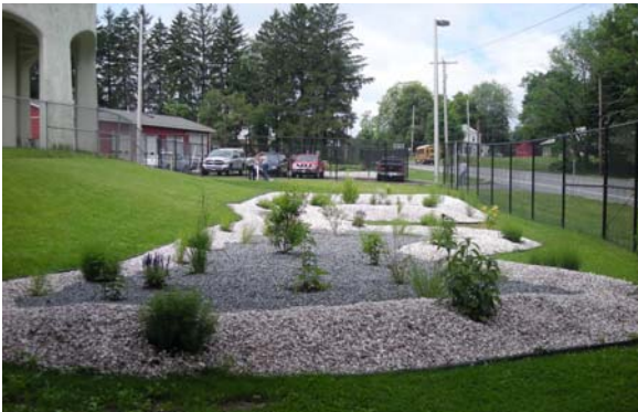
Soil & Water District staff designed and assisted Treatment Plant staff with planting shrubs in this completed rain garden at the Water Treatment Plant in Newburgh, NY. The Water Department staff built the rain garden.
