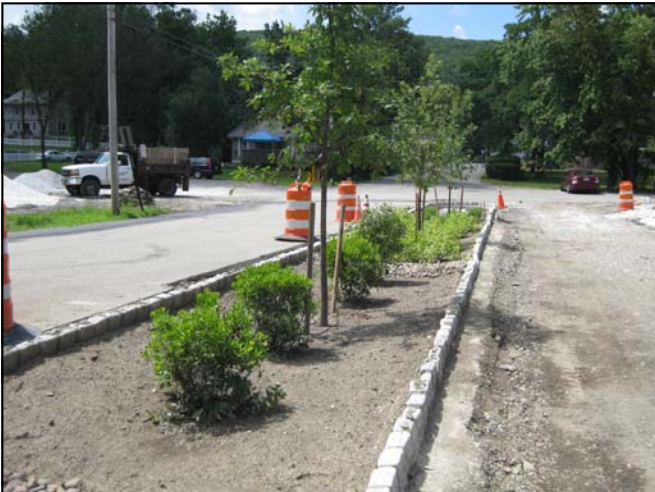
The vegetated swale is in place.
