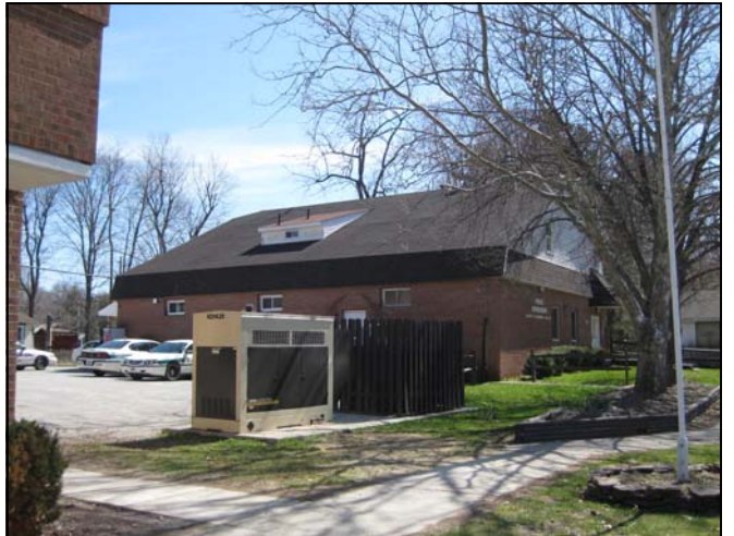
The "Before" photo shows a generator and dumpster—they have since been moved. The generator is by the Police Department and the dumpster is now to the side of Village Hall.
