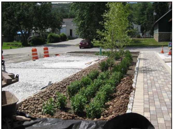
The rain garden is located right in front of Village Hall and the pervious paver sidewalk.
