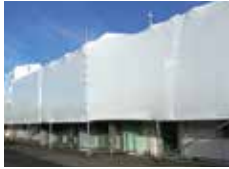
• Scaffold or Containment Shrink Wrap
