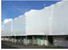
• Scaffold or Containment Shrink Wrap
