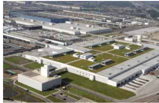
Living roof composed of sedum growing on top of the Ford Dearborn Truck Plant final assembly building
