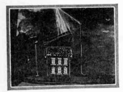
A model of a house is exposed to a Tesla coil discharge to simulate lightning. A little aerial protects it, and no harm is done.
