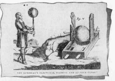
Here the primitive frictional electric machine with no multiplying gear is shown, and the experimenter, carrying an excited ball of sulphur, is driving a feather about through the air. The Experimenter for November, 1924
