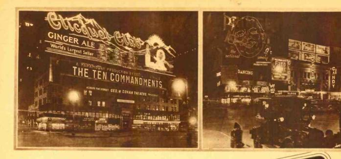
There is plenty of "ginger" in the largest electric sign on Broadway that achieves its effects at the cost of 19,000 lamps supplied through 21 miles of wire and with the consumption of over 300 horsepower. It is over 200 feet long. The jovial smoker of Prince Albert tobacco at the right is burning 2,775 electric lamps and using about 60 horsepower.
