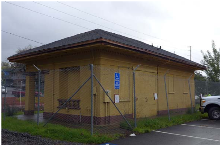
Figure 5. The north and west elevations.
