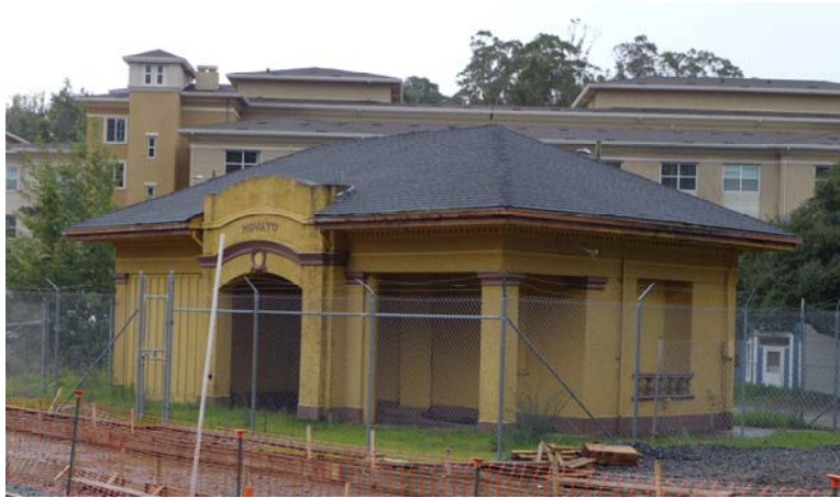
Figure 25. The hipped roof.
