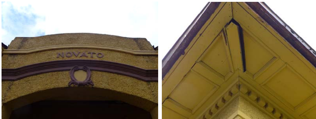
Figures 9 and 10. The entryway decoration (left); dentils and paneled soffits of the roof. (right).
