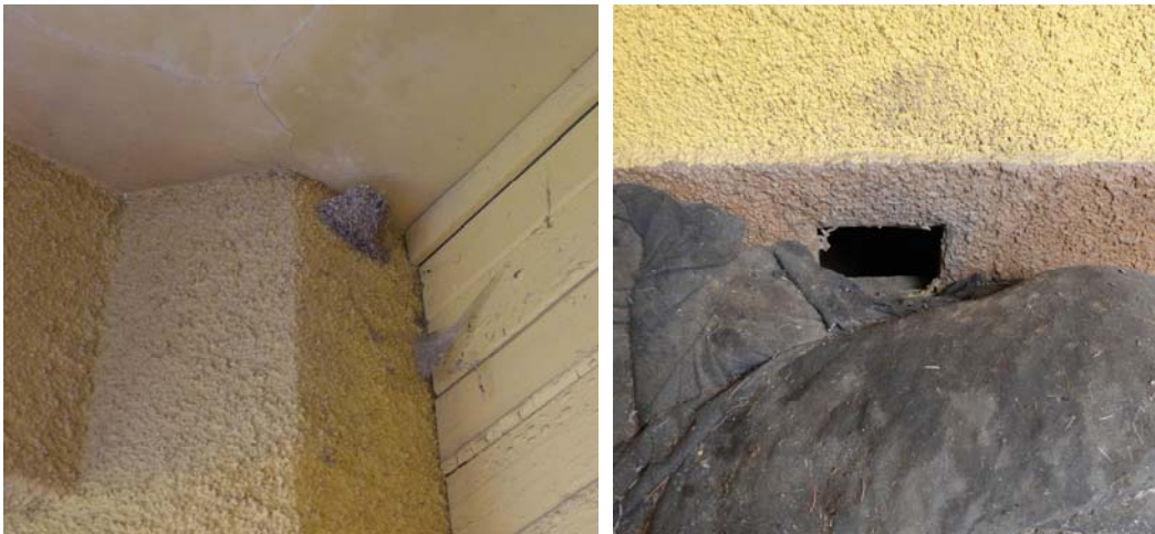
Figures 39 and 40. Bird's nest under the walkway (left) and the open vent (right).
