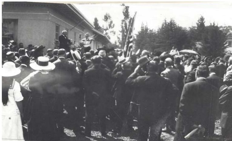
Figure 19. The existing depot, on the dedication day in 1917; see west elevation windows behind the speaker. Novato History Museum.
