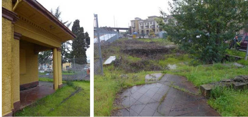
Figures 7 and 8. The waiting shelter (left); the concrete paving and the foundation remains (right).
