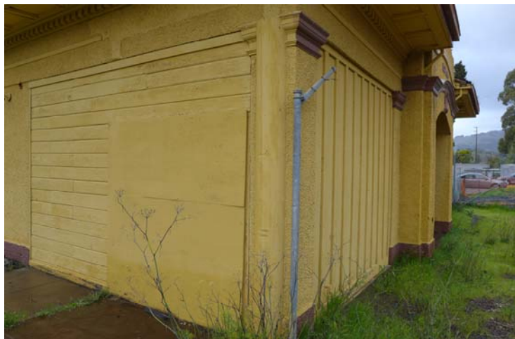
Figure 31. Wood siding at the southeast corner.
