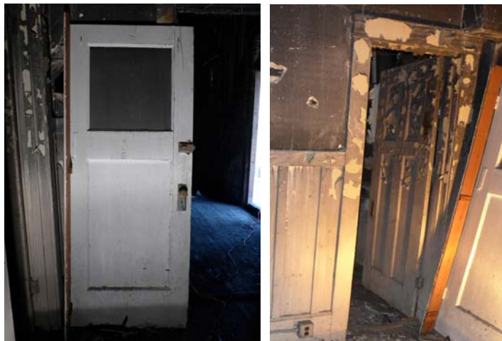
Figures 49 and 50. Existing interior doors.
