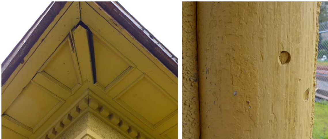
Figures 34 and 35. Cornice paneling (left) and semi-circular timber (right).
