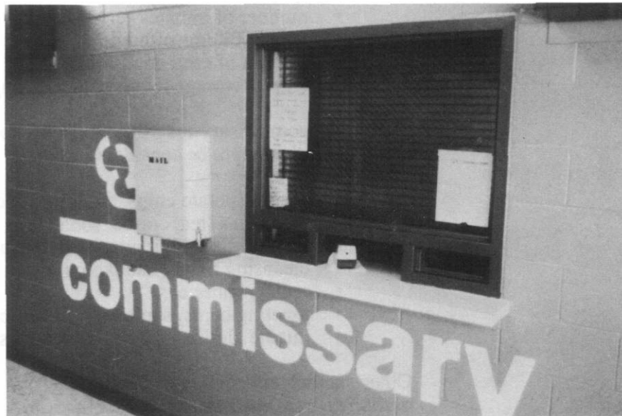
Commissary pass-through window located on main jail corridor.
