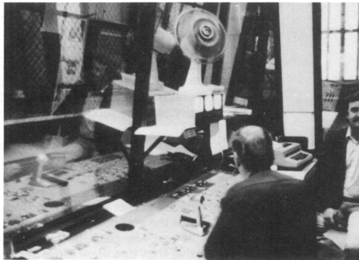
Reflective glass in the control center can inhibit officer view when light levels are too high in the control space.
