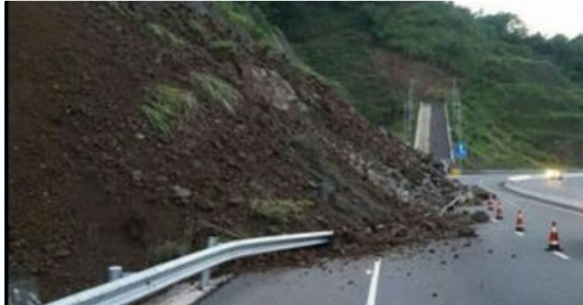
Landslide on Mount Rosser Bypass
