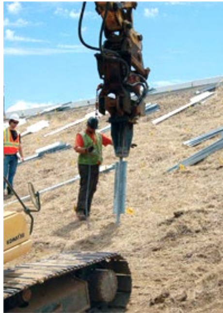
Figure 3. Platepile installation (McCormick 2014).
