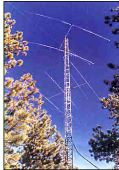
The 90-foot tower, complete with a 40-meter beam and a Cushcraft A-4.
