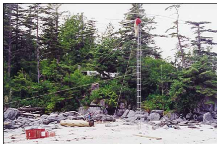
Terry, VE7TLL, at the top of one of the 30-foot towers, working on one of the tri-banders.
