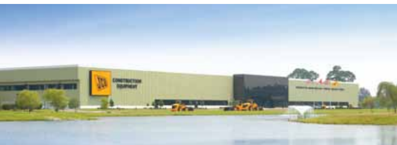
Built in 2000, the JCB North American Headquarters in Savannah, Georgia supports all United States and Canadian dealers and manufactures the world's safest skid steer and compact tracked loader.
