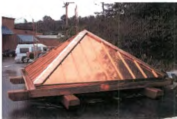
Copper roof section, prior to installation
