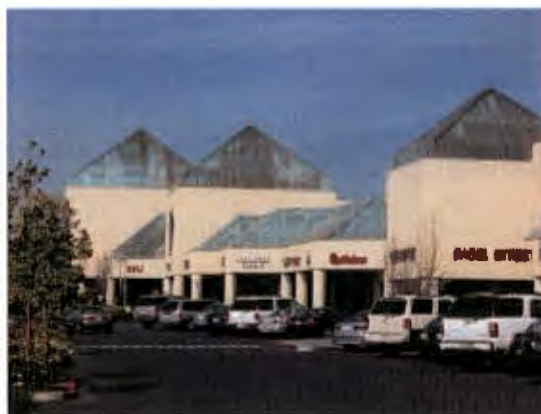
Copper roof, Redwood Shores California
