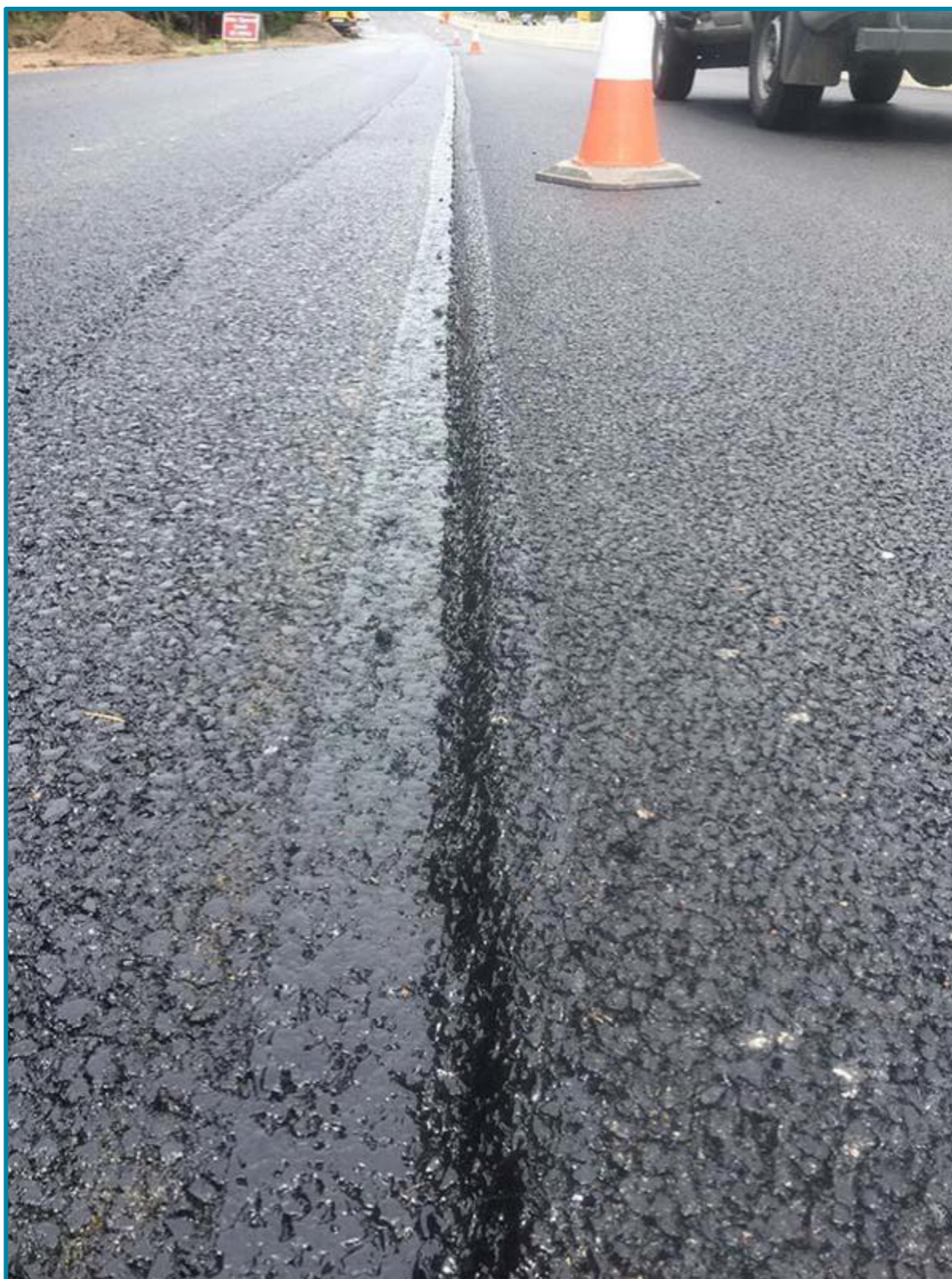
Figure 12 County Council Innovation Scheme Trials of 30° Chamfered Cutting Wheel- Painted Joint (provided by an MPA member)
