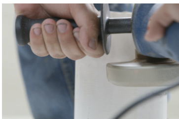
1. Abrade & Clean the substrate
