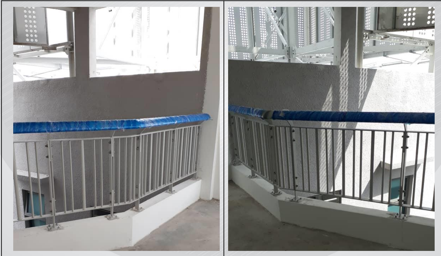
Railing at rooftop installed.
