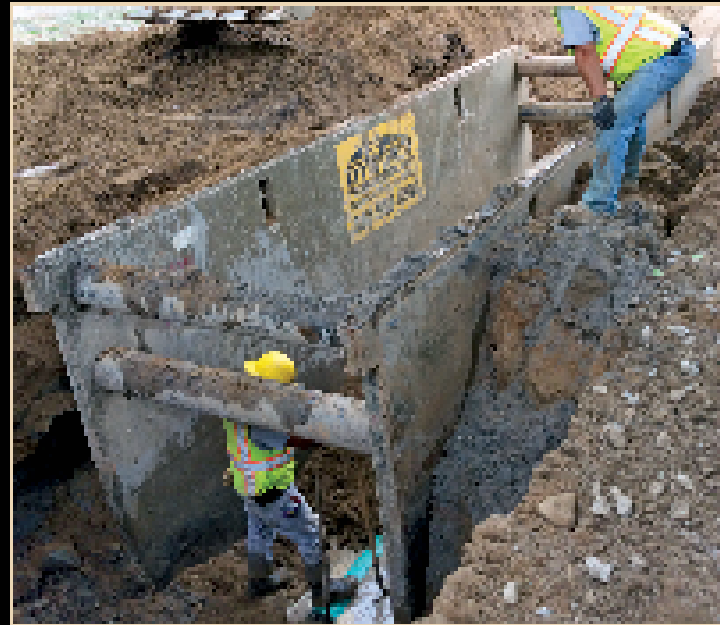
Steel Trench Shields
