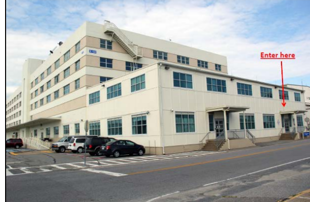
JECC Hdqtrs Bldg X 132 9712 Virginia Ave
