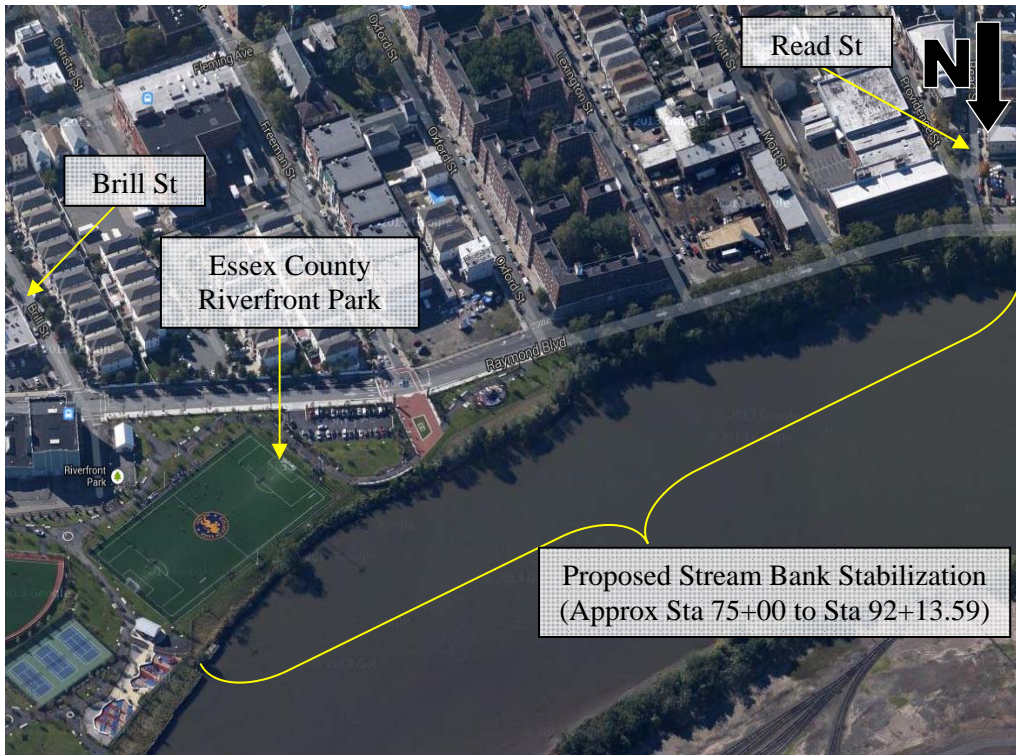
Figure 5: Aerial View of the Stream Bank Stabilization Project Area, Station 75+00 to Station 92+13.59 (End Section)
