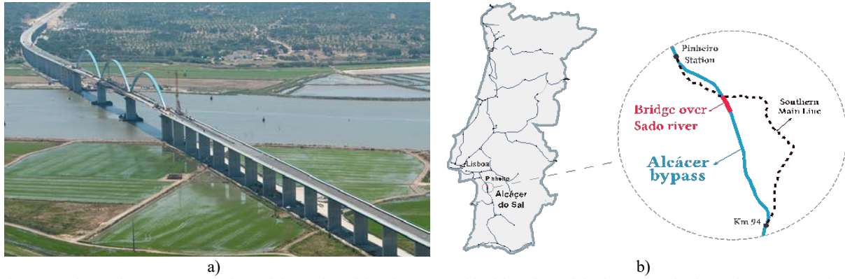
Figure 1. Alcácer bypass: a) overview of the Sado Bridge, b) geographical location of the bypass and schematic representation adapted from REFER [33].
