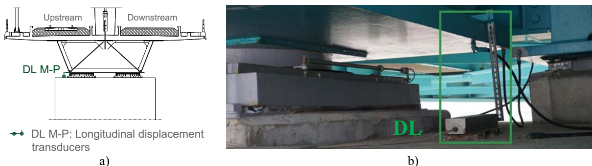
Figure 11. Longitudinal displacement transducer (DL): a) cross section location, b) sensor installation.
