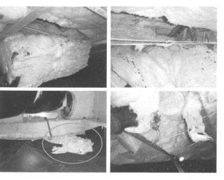
I saw a burrow hole under the foundation. This is at least one spot from where the rodents could be entering.
