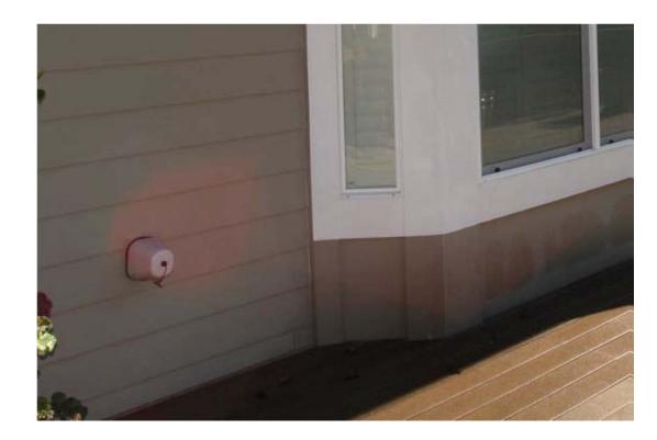
106. If installed, the flashing allows water to escape from behind the siding onto the deck while also preventing water from making its way down into the deck-to-wall joint, where it can cause rot. That z-flashing is required if the deck is not built at least two inches below the siding, as required by the building code, the siding manufacturer, and standard good building practice:
