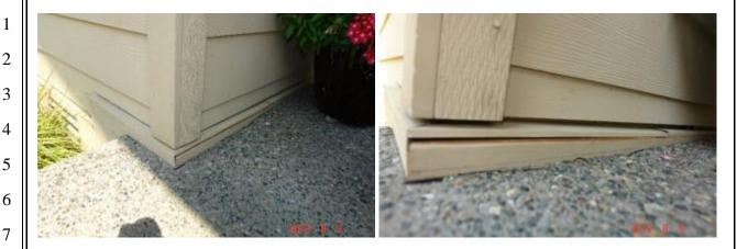
96. And Shea's failure to install an L-metal flashing also means that water makes its way down between the patios and the wood, which leads to damage such as at this Trilogy home:
