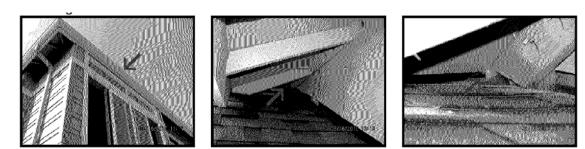
There are openings at the intersection between the overhang and the roof on the west side of the entry through which birds and rodents can enter into the attic. These openings should be covered with wood, wire mesh or filled with aerosol foam.
