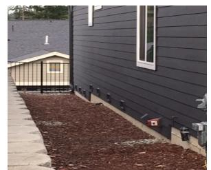
The above photograph shows crawlspace vents along just one elevation of at recently built Trilogy home:
