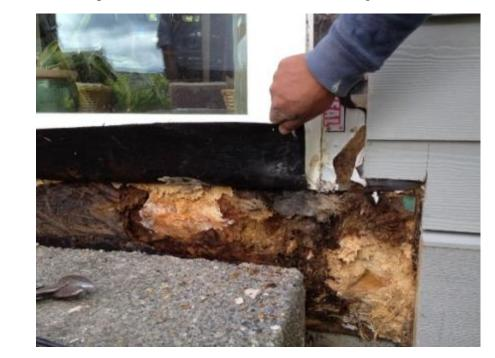
97. As with corbels, knee braces, and columns, Shea replaced damaged wood due to missing patio-to-wall flashing on one of its own model homes before selling it.
