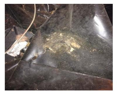
144. Rodent's feeding habits are destructive, and their nesting behaviors can compromise the structure of infested homes. Rodents destroy insulation, electrical wiring,
