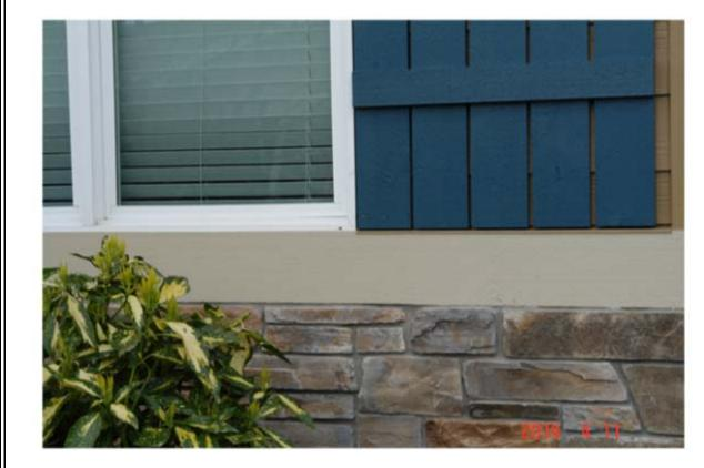
100. The architect's drawings approved by King County required the installation of a flashing at the wainscoting:
