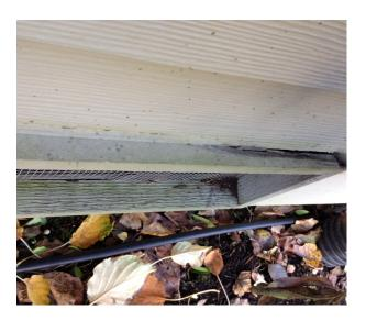
148. Shea also failed to install an adequate number of vents on many homes. And even with extensive venting, Shea still had to install crawl space vent fans to try to increase circulation
