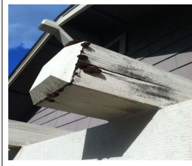
67. An internal Shea document recently obtained shows that in August 2009, Shea calculated its "Exposure by Plan" for each of the home plans (models) at Trilogy based on its omission of the flashing from the corbels and knee braces. Shea calculated that the cost of replacing those components on the 671 homes that it had built by that time was in excess of \$1.4 million.
