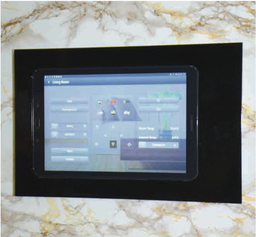
WS Retrofit into stone with Samsung
