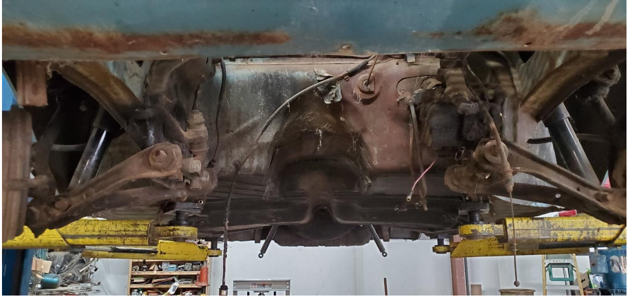
Empty hole from below.
