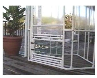
Add two 23 1/2" poles horizontally and another 10 1/4" [N] pole, connect with two 90 degree corner connectors, and adjust everything for a nice snug fit.
