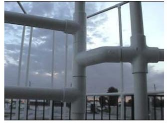
The final step is to make two bars that will fill in the space above and below the door. These bars are made with pvc poles cut to [M] length and capped with oversized T connectors (1x1x3/4) that have been trimmed to fit. (One alternative option is to trim a couple of pieces of plastic gutter guards to fill the openings around the door).
