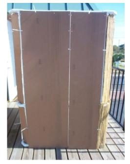
Drill from the shiny side to make holes approximately every 6" to 12", (which are for cable ties to attach the panel to the cage frame.)
