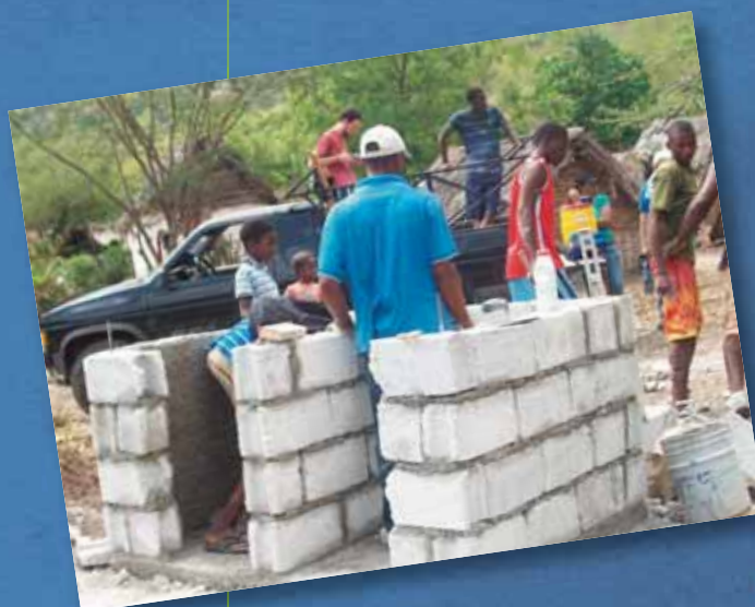
2nd composting toilet: view of vaults under construction, teammates on truck in background
