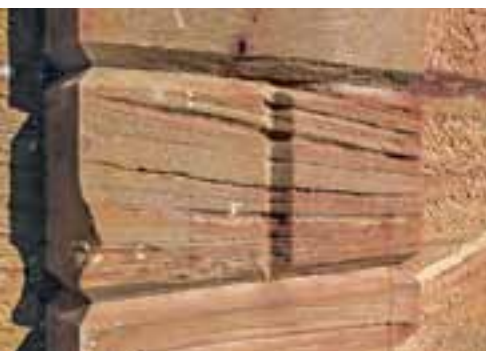
Sandstone building stone used in the wall of the hunting lodge at Chatelherault, near Hamilton. © Lorne Gill/SNH
