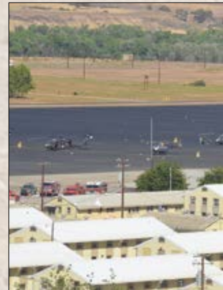
The newly surfaced Camp Roberts helipad is used by California National Guard helicopters during annual training. Photo by Capt. Jason Sweeney
