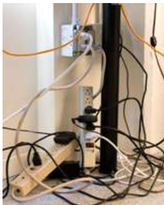
Overloaded circuits
