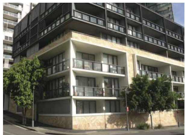
Photo K2-9 Example of a building that strongly defines the street corner and street edge
