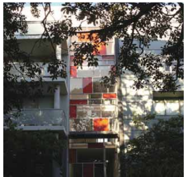
Photo K2-19 Building entries can be distinguished through the use of colour, as well as awnings that extend into the public domain
