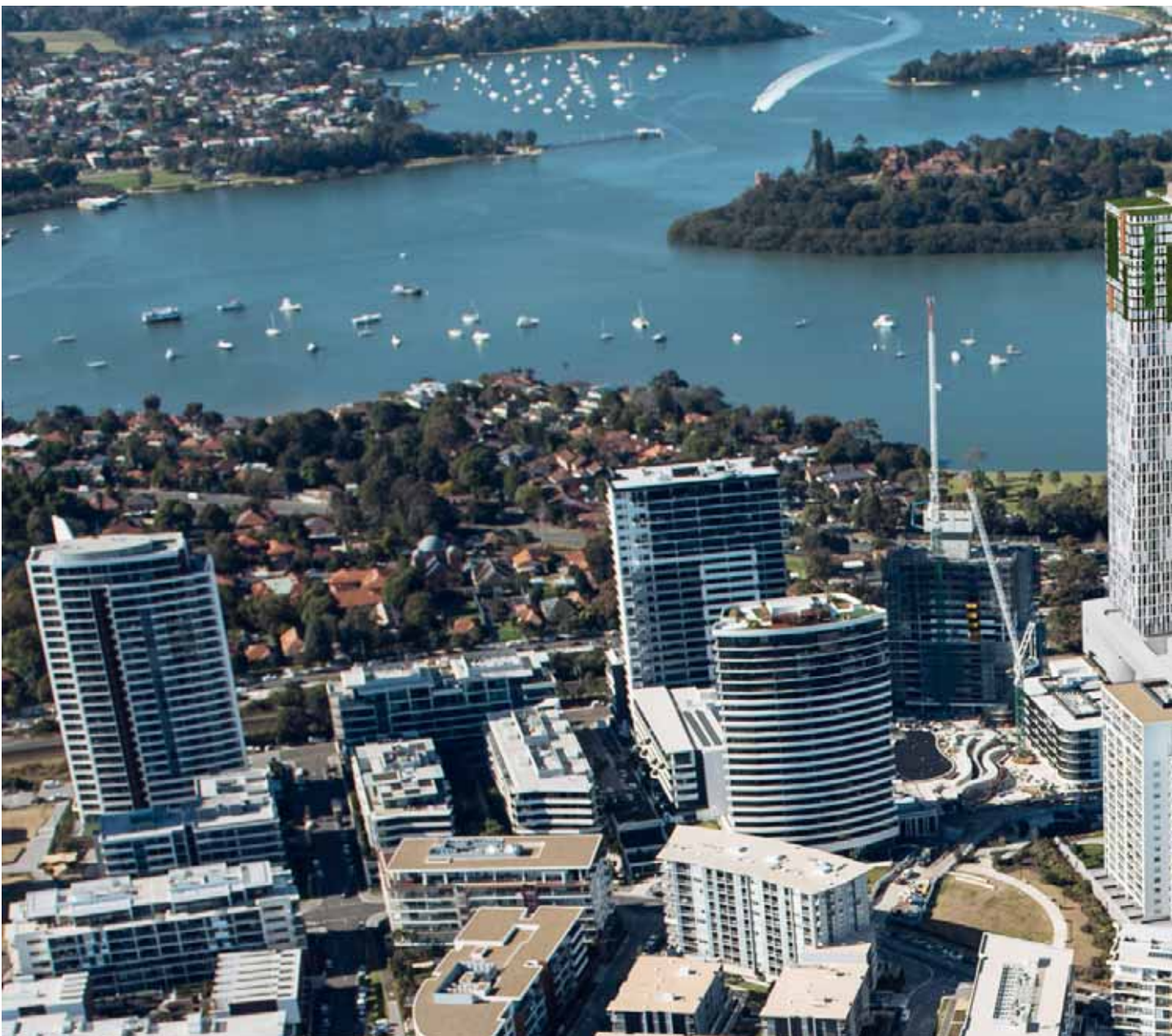
Figure K2-35 Indicative Development Concept Not to scale. The diagram illustrates the indicative concepts for built form and public domain
