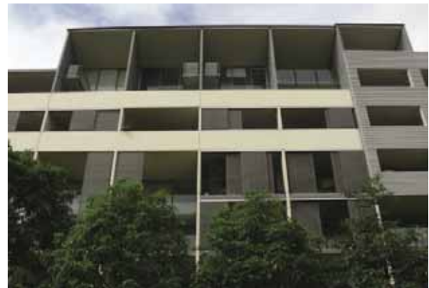
Photo K2-17 Deep balconies and adjustable screens shade windows from undesirable heat gain
