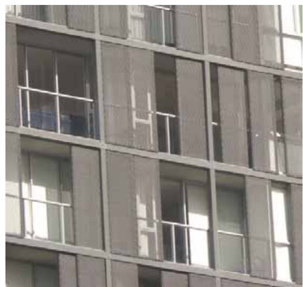
Photo K2-18 Using one type of sun shade over large areas can add to building bulk
