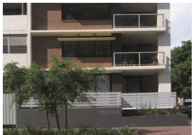
Photo K2-28 Front fences have some transparent quality to allow for surveillance of the adjoining public domain, we well as privacy for occupants
