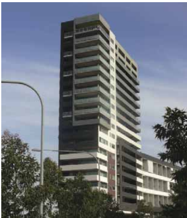
Photo K2-7 Variety in building types is required on large sites
