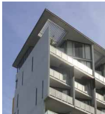
Photo K2-13 Roof form adds to building articulation
