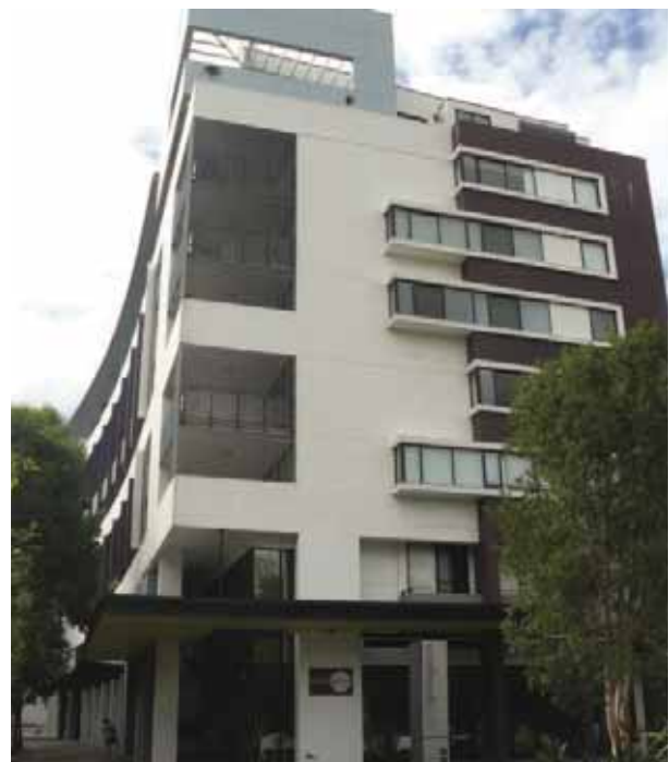
Photo K2-8 Well articulated facades including refinement in window and balcony design
