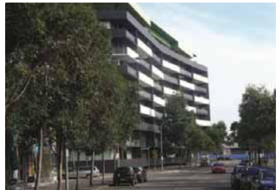
Photo K2-14 Principle of curved street geometry reflected in building form suitable for Shoreline Drive
