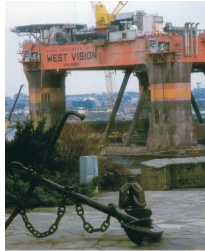
Cable distribution cabinet on an oil drilling Stavanger, Norway.
