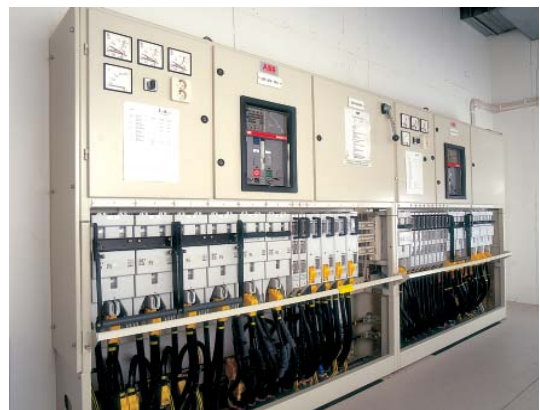
Safe switchgear with busbars and devices, Kabeldon IP-system.
