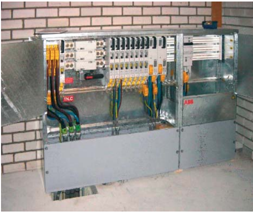
Distribution board 1600 A at an industry.
