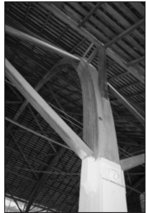
Hewins Park Pavilion has been a centerpiece of community activity in Cedar Vale for nearly a century. (Right) Six laminated radial arches anchored by concrete bases support the gabled roof.
