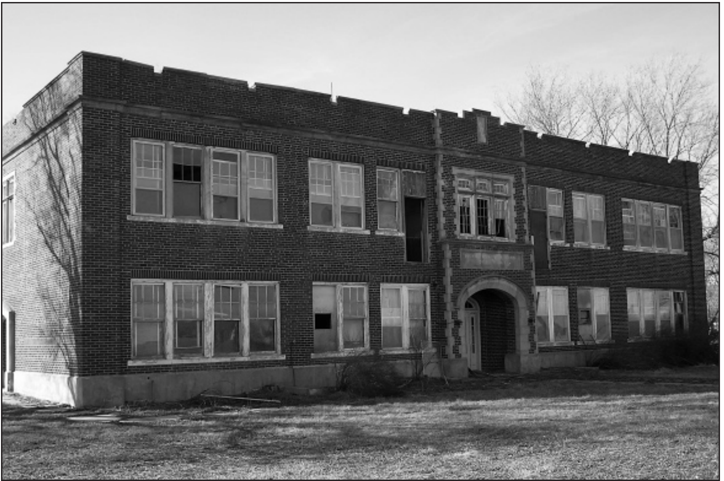
Vacant since 1989, the former Mahaska High School building in Washington County is being renovated for use as residences.
