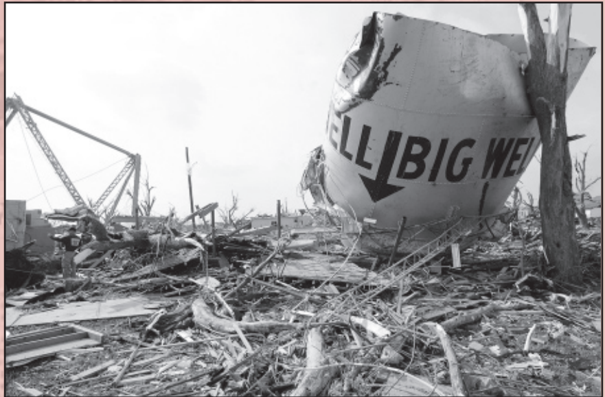
While the Greensburg Well itself was not severely damaged, the buildings atop the well were destroyed. Photo courtesy of The Wichita Eagle/Kansas.com.
