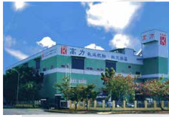
Kaohsiung Taiwan Plant
