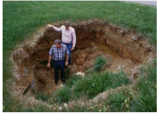
Figure 8. A collapse sinkhole in Knox County, where thicker residual soil covers limestone (highway right-of-way, I-75).
