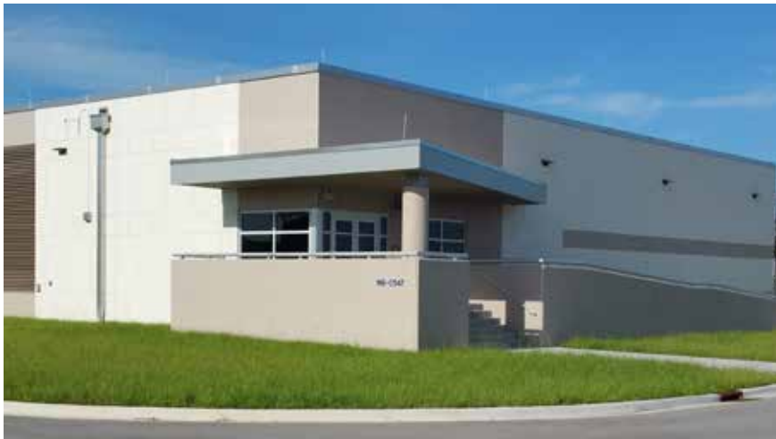
The Data Center Consolidation Project at KSC has successfully migrated three less efficient Data Centers into a new power efficient and more reliable Data Center Facility.
